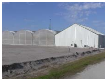
Figure 1. The Harris Moran Seed Company's Research Station comprises a laboratory, offices, 12 greenhouses and several acres of cropland. Years of research & development results were threatened due to a poor electrical grounding system.
