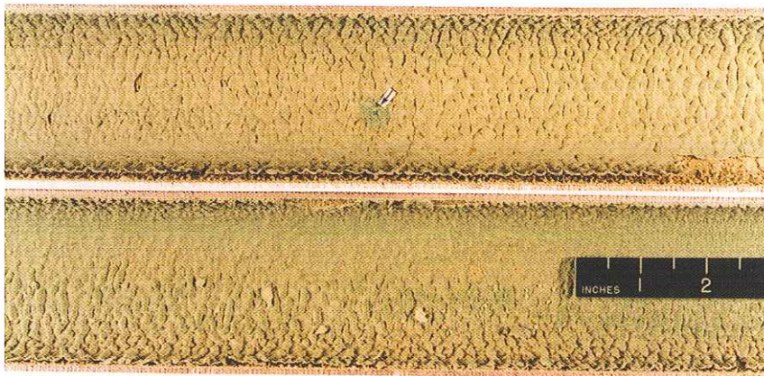
PHOTO I. A tube-wall perforation (see arrow) covered with a friable tubercle of green copper-corrosion products. The cupric oxide on the tube surface is covered with a relatively thick, loosely adherent layer of brown deposits from the hot water conveyed. EDS will reveal that the deposits contain significant amounts of aluminum.
