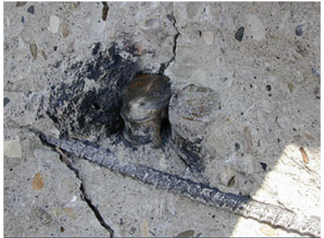
FIGURE 5. Burn scar on shattered concrete is evidence that lightning found a vertical reinforcing rod (center), which likely acted as an efficient Ufer ground, offering lower resistance than that of the installed grounding/lightning protection system.
