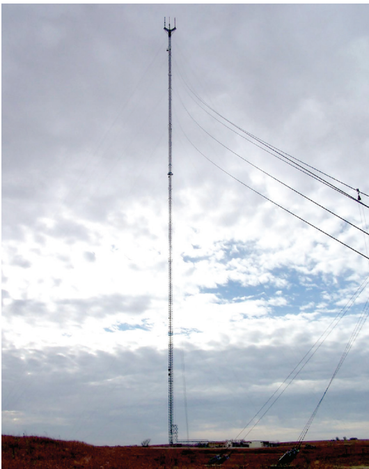
A robust, low resistance ground system renovation solved many lightning created problems plaguing this 2000-ft TV tower.
